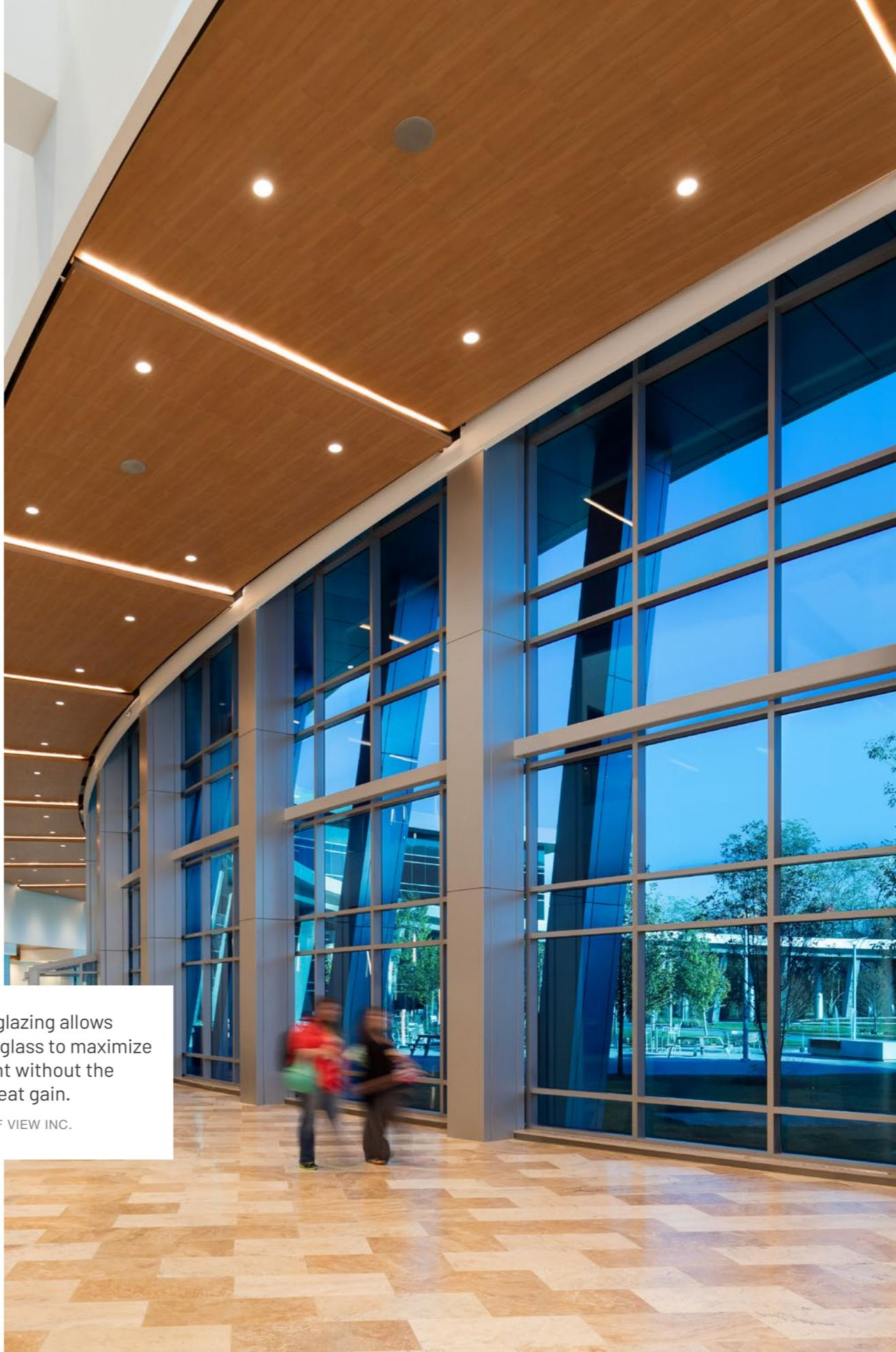
Electrochromic glazing allows extensive use of glass to maximize access to daylight without the corresponding heat gain.
