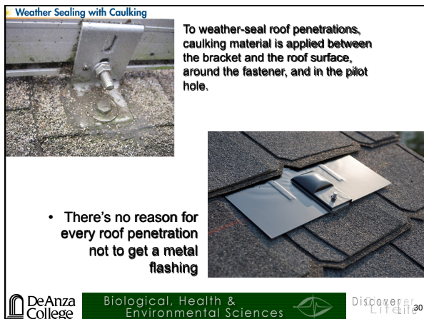
Weather Sealing with Caulking
