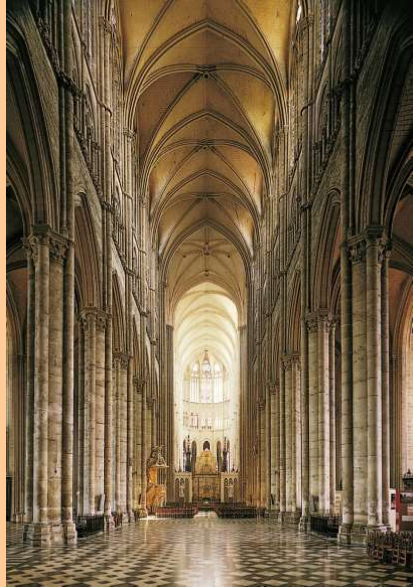
ROBERT DE LUZARCHES, THOMAS DE CORMONT, and RENAUD DE CORMONT , interior of Amiens Cathedral (looking east), Amiens, France, begun 1220.
