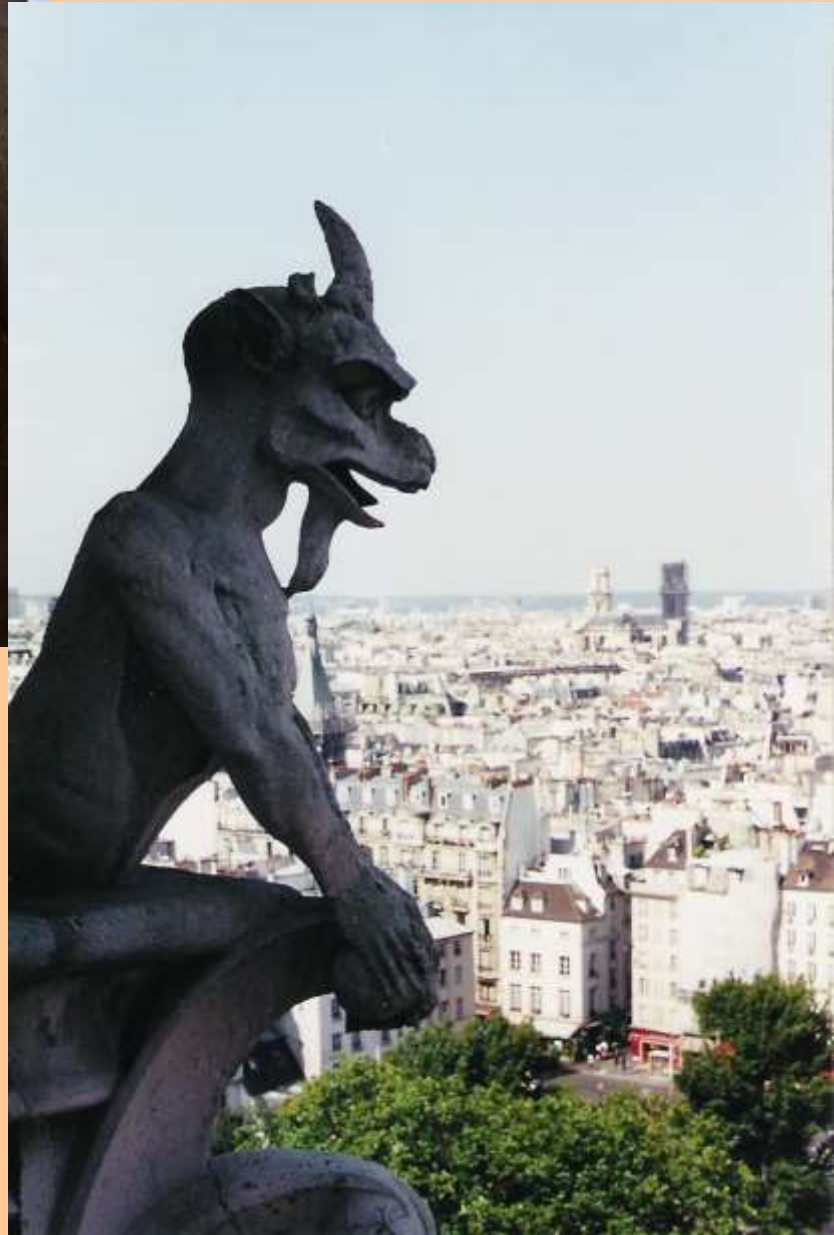
Gargoyles at Notre Dame Paris, France, begun 1163 (serve as drain pipes as well as decorations.)
