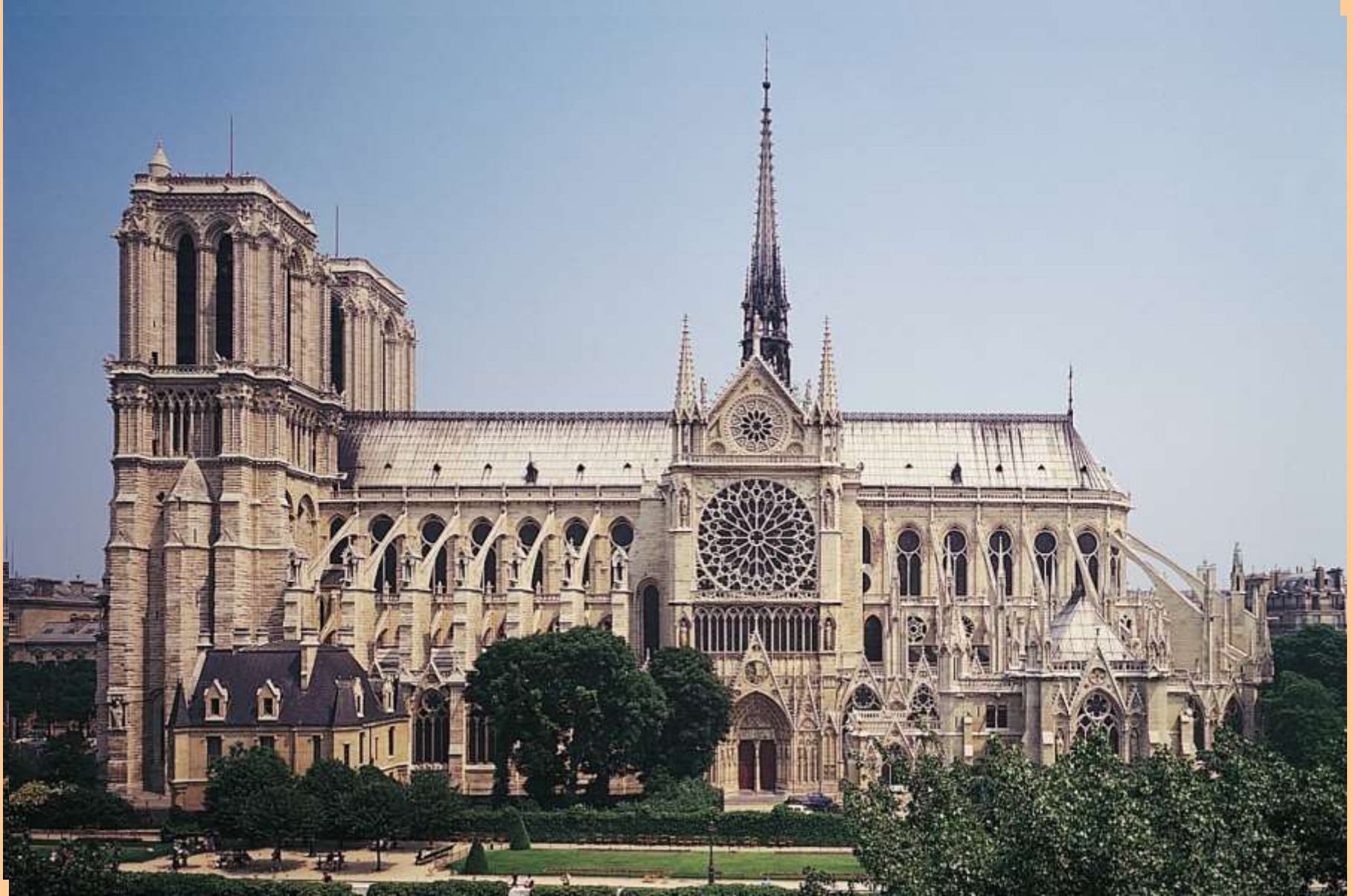
Notre-Dame (looking north), Paris, France, begun 1163; nave and flying buttresses, ca. 1180–1200; remodeled after 1225. It was among the first buildings in the world to use the flying buttresses
